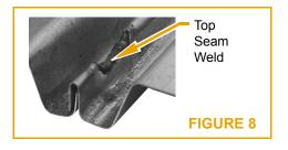
Top Seam Welds: When sidelaps of FORMLOK decks are connected with top seam welds (TSW) (Figure 8), the 1½ in. long weld must engage the top of the inner (male) leg. Clinch the joint before welding to create positive contact between the lips.
